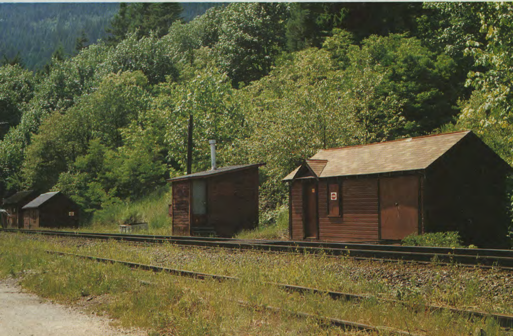
(Below) This view of the CPR buildings at Yale in July 1984 was taken from almost the same position as the one above.
