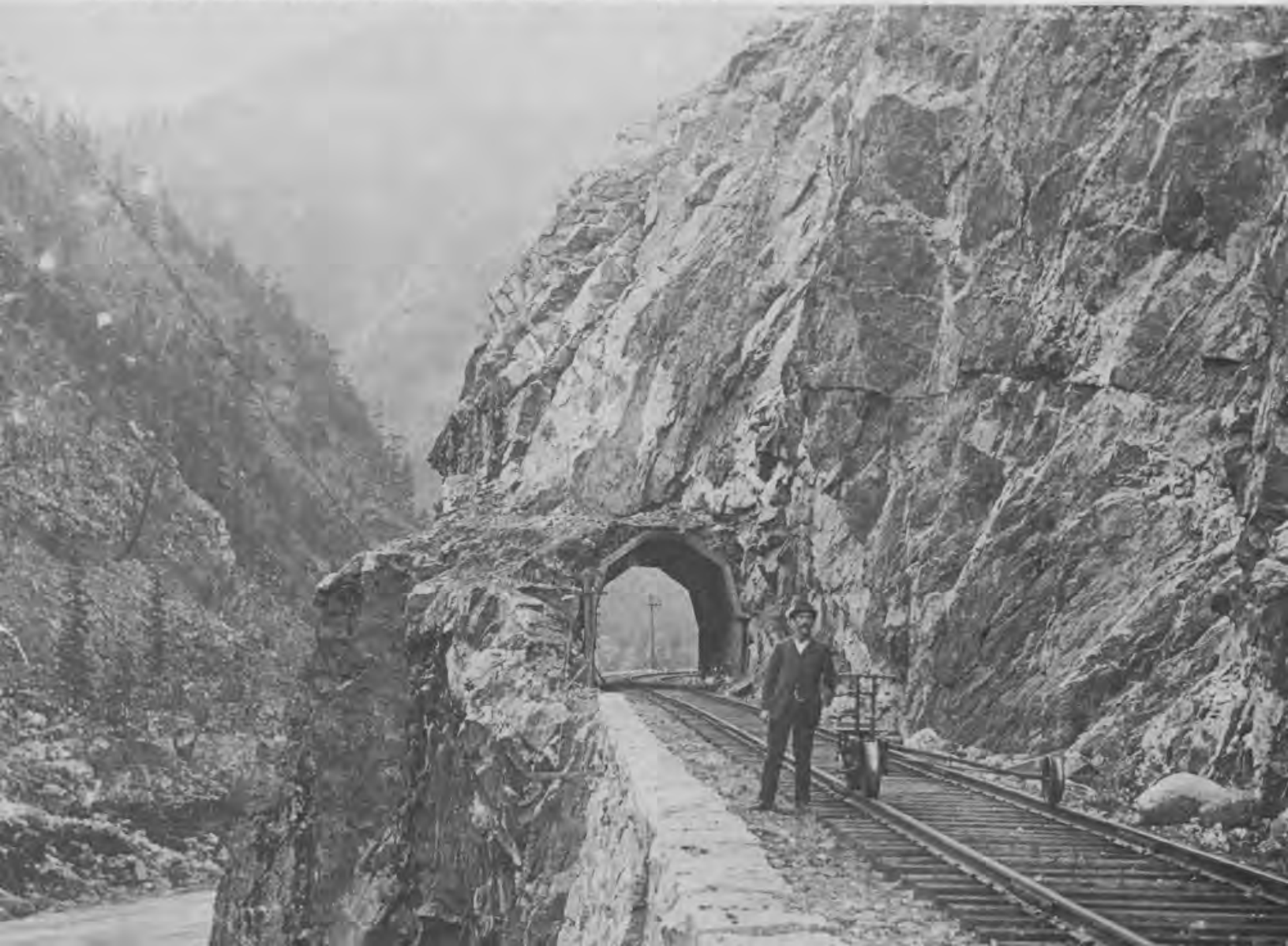
Cariboo Joe's Tunnel, CPR, in the Fraser Canyon. Note the masonry walls.
