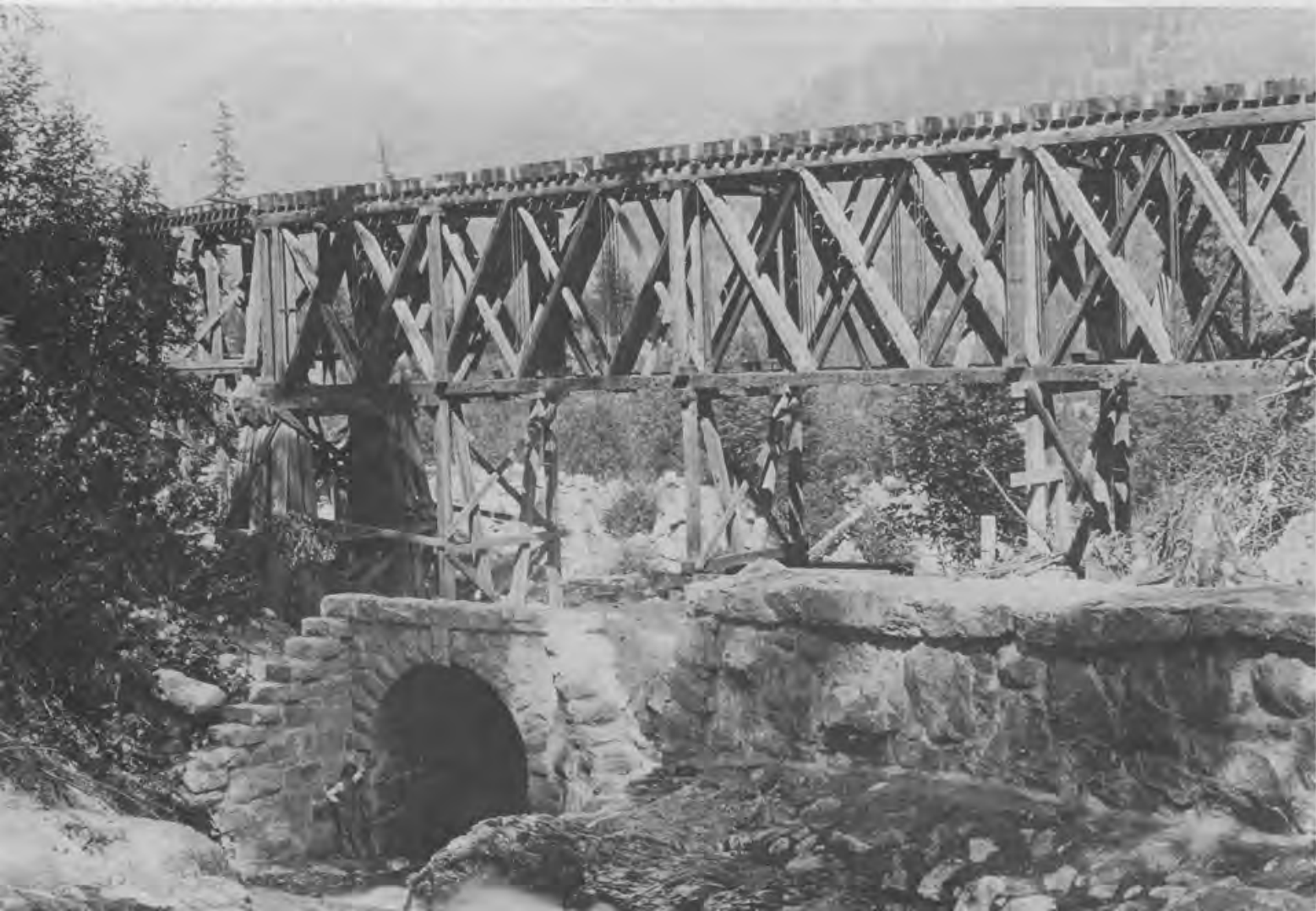
The Quoi Eck trestle and replacement culvert, four miles east of North Bend. Note the masonry work.
