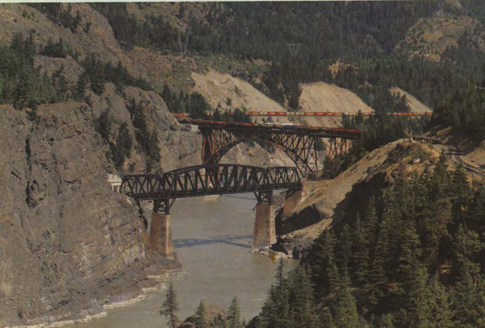
(Below) Railroad bridges at the site of Cisco in August 1985. The black bridge in foreground sits on the original piers of the cantilever bridge shown above. The original cantilever is still in daily use on Vancouver Island, where it was re-erected. Second bridge is the CNR bridge.
